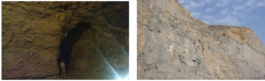
Figure2. Geological survey at preconstruction stage on autcrops and slopes (right) at construction stage in tunnel route (left) [8]
