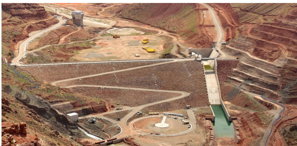
Fig. 2. Downstream view of Vanyar Dam at the end of construction
